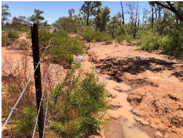
Photo. Eroded fence line
